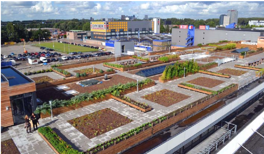
The rooftop farm of Zuidpark can be used both for lunch and for corporate events.
