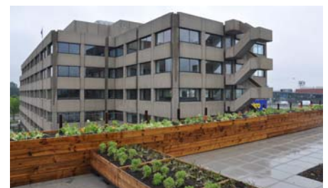
The green roof can be seen perfectly from the offices of the higher opposing building - a welcome change in an area predominated by industrial buildings.
